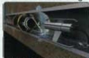
Leaking joint in mainline sewer
