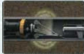
Grout collar stops infiltration
