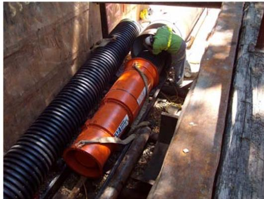
**Figure 6: OSHA Approved Ventilation Equipment w/ Corrugated HDPE Ducts**
