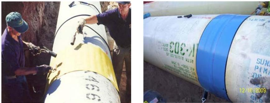
**Figures 3 a, b: Application of a Heat Shrink Sleeve, Completed Joint per AWWA C216**
