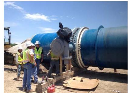
Figures 3a, b, c: Trenching, Pipe Laying, Butterfly Valve Installation in Section C, STA 2404+15
