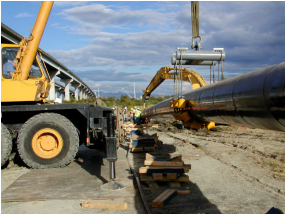
Figure 7. Entrance of 36 in. pipe at Swinomish Channel
