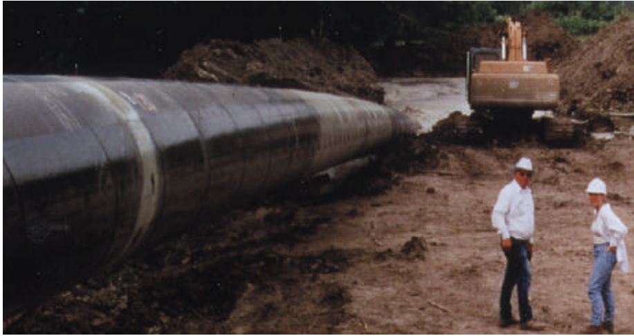
Figure 4. Entrance of 48 in. pipe at Guadalupe River Crossing.
