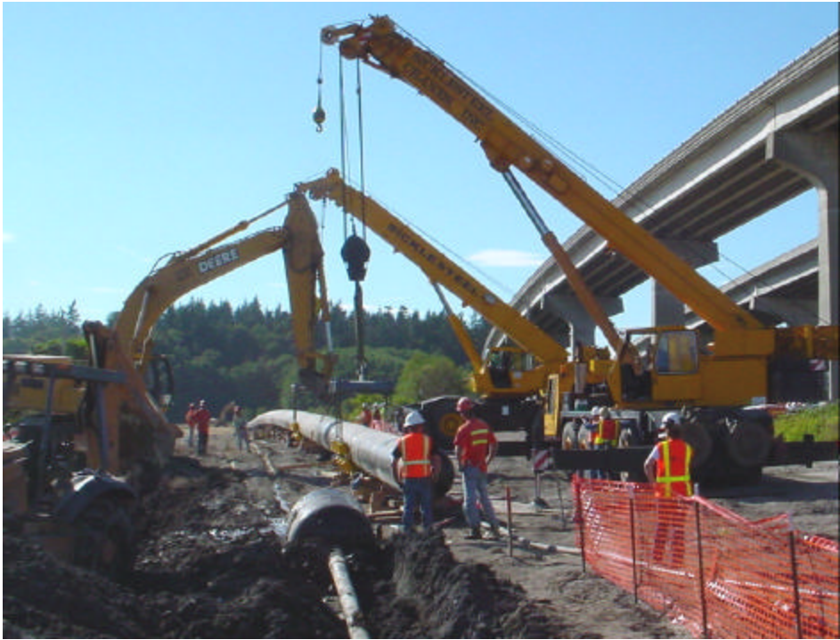
Figure 6. Preparing for pullback of prewelded 36 in. pipe
