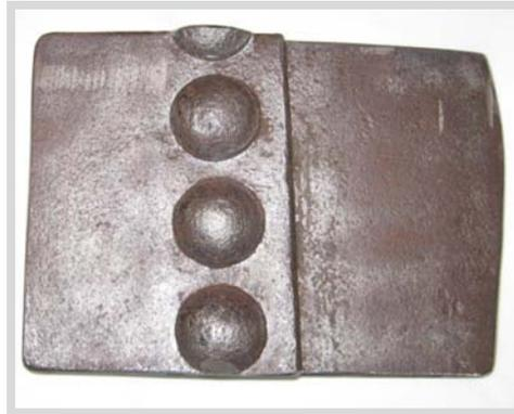
**Figure 1 : Riveted Steel Pipe Joint**
