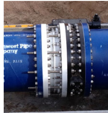
Figure 2: Dismantling Joint Restrained with Tie Rods Connected Through Adjoining Flanges.
