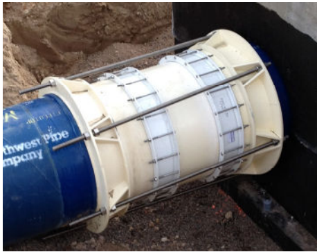
Figure 1: Paired Harnessed Mechanical Couplings at Structure
