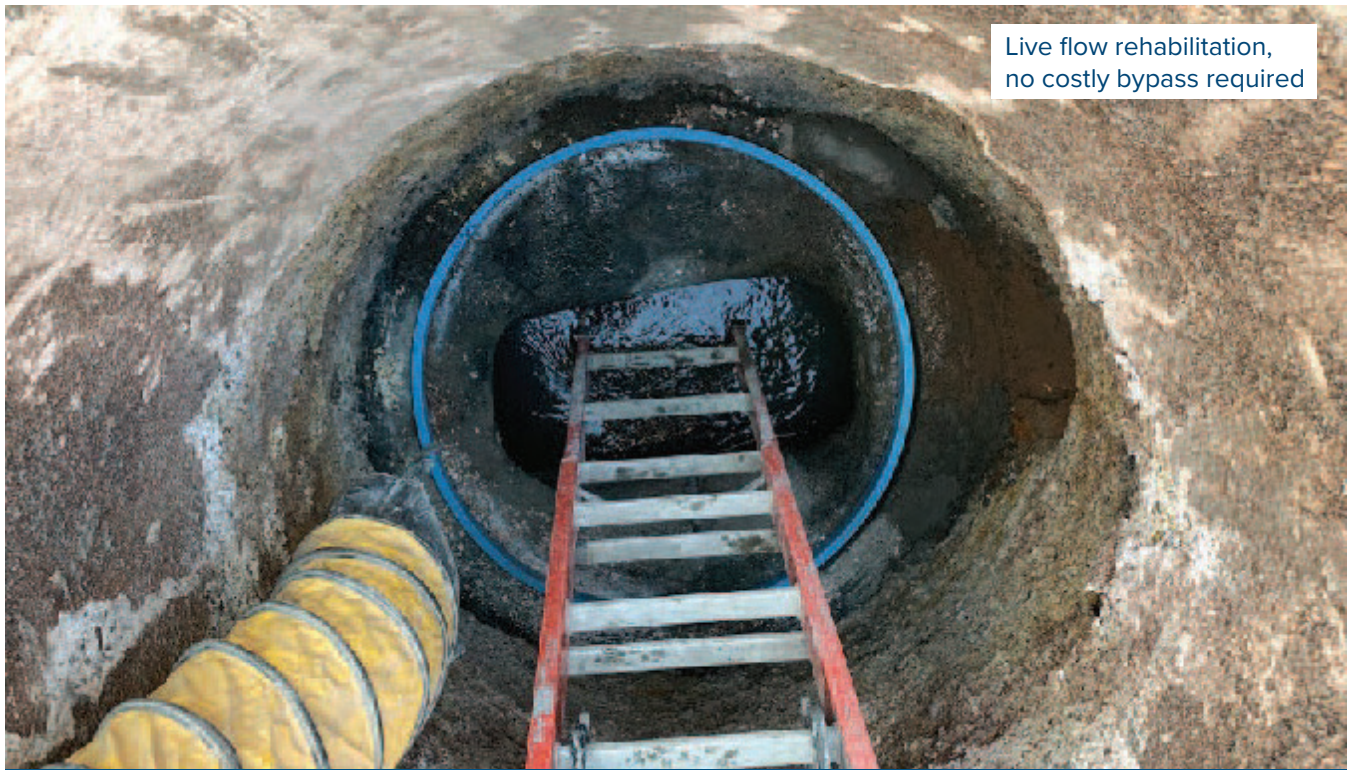
Assuring the riser fit the rebuilt bench
