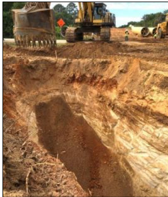
Figure 3: Trench Cut in Sandy Soil
