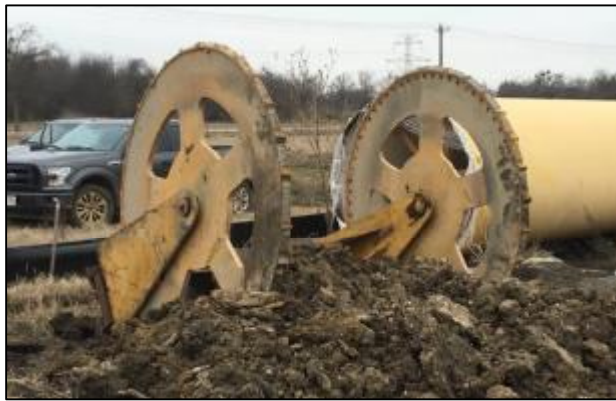
Figure 5: Wheel Compactor for Granular Embedment
