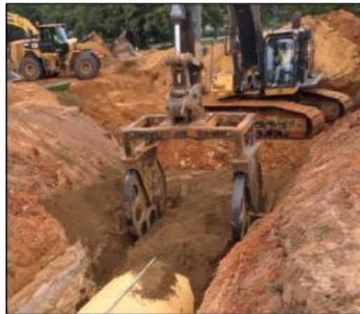
Figure 9: CSS Being Compacted with Roller
