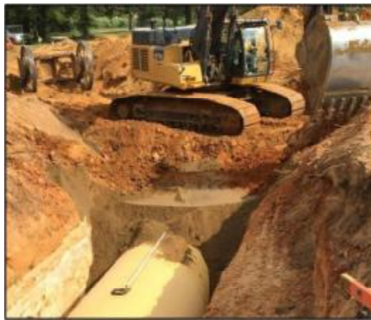
Figure 10: CSS Compaction Completed
