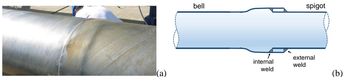
**Figure 1. Configuration of lap-welded steel pipe joint.**
