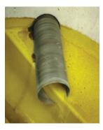
Establish the alignment and elevation of the new connection that is to be made. Core an opening through the outside of the manhole into the main channel. It is recommended to make the opening 2" larger than the OD of the new connecting pipeline. Coring bit should be long enough to reach the main channel (be ½ the inside diameter of the manhole plus the manhole wall thickness.) If a coring machine is unavailable, create a rough core using a grinder with a masonry blade and a roto hammer.
