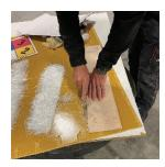
Measure the area of the grout to be covered and add  $\chi''$  per side. Mark and cut the woven FRP sheeting to size. It is recommended to cut the FRP sheet into four separate pieces.
