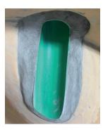
Inset the PVC pipe into the manhole and place a spacer under the pipe to create a consistent flow line and create as annular space for the grout. On the inside end of the manhole shelf place a piece of cardboard against the channel and secure it with duct tape to dam the ends of the cavity for grout. Install the boot on the outside of the manhole. On the inside of the manhole pack grout around the PVC pipe and finish the top of the grout with a damp sponge. Allow the grout to dry.
