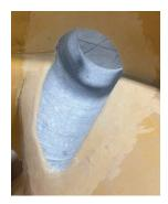
Using an Angle grinder with an abrasion wheel, abrade a 2" width of the FRP manhole on the bench shelf along the edges and above the core drilled pipe channel.
