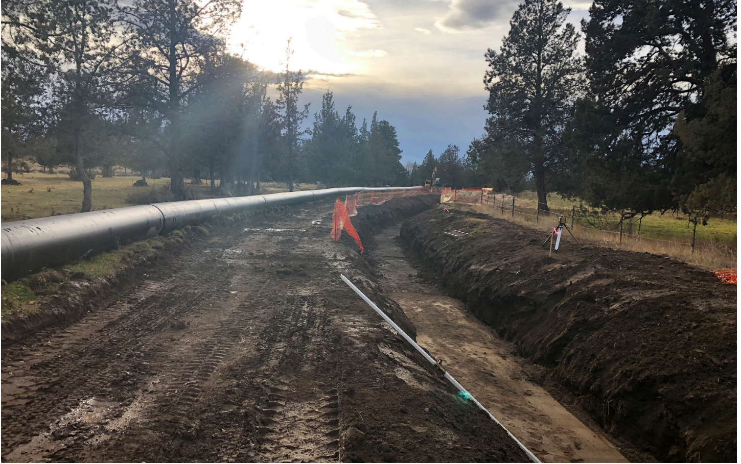
Work on phase 1 of the Pilot Butte Canal piping project.
