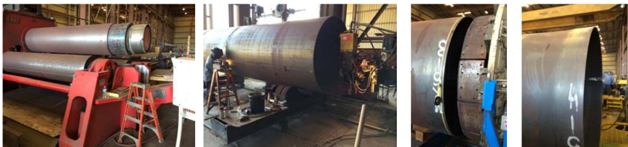
Figures 5a, b, c, d: Pyramid-type Rollers for Plate Rolling, Girth-seam Welding of two Sections of Reliner, Hydraulic Expander for Belling, Completed Bell
