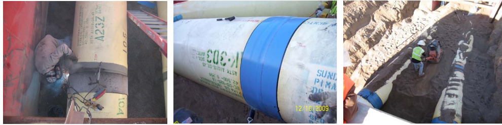
Figure 3a, b, c: Joint Welding, Heat Shrink Sleeve Installation, Backfill Compaction
