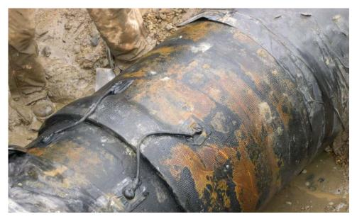
Figure 3. Ductile Iron Pipe Bonded Joint (Southwest Pipeline, 2004)
