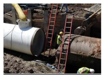
Figure 2. 1906 72" Steel Pipe connected to new Steel Pipe in NJ (National Welding Corporation, 2006)
