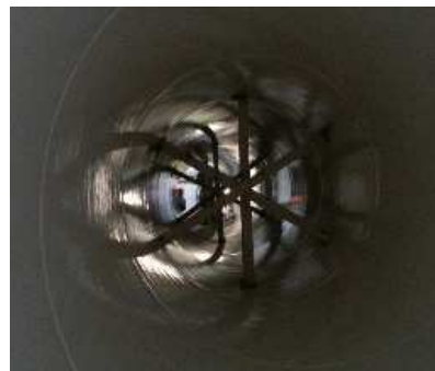
Figure 10: Two inside stull sets are visible
