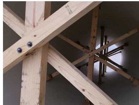
Figure 15: 5 sets of a 3-stull spider configuration
