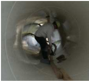
Figure 7: The Vertical stull is fit into place
