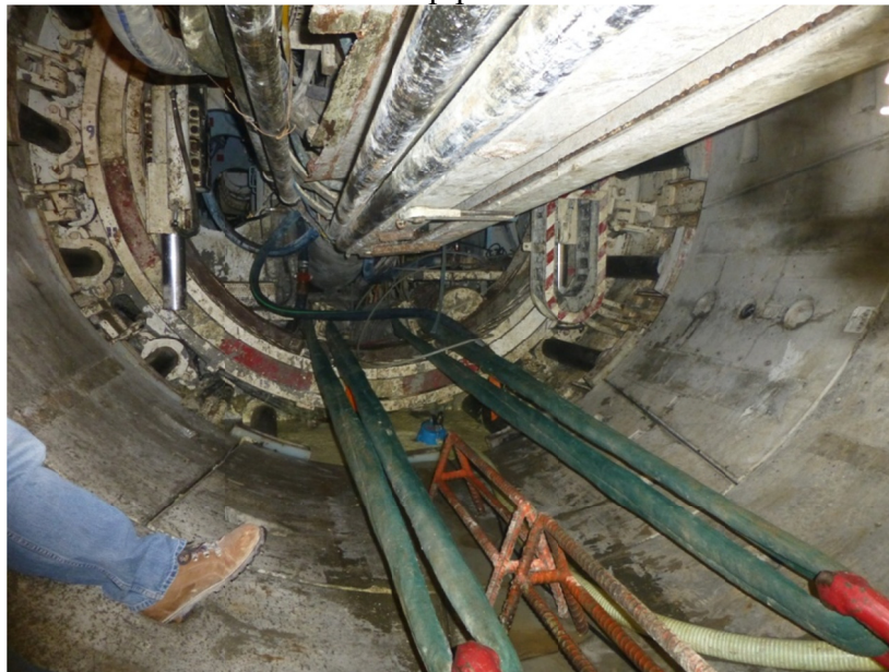
Figure 3. TBM leaves 10 foot diameter segmented tunnel
