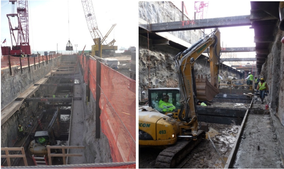
Figures 2a and 2b. Launch Shaft excavation.
