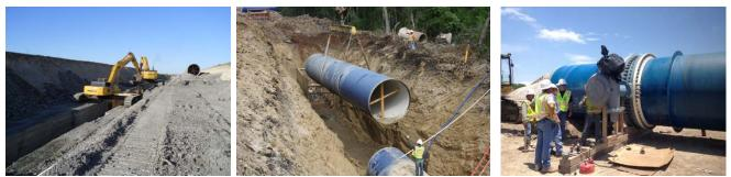
Figures 3a, b, c: Trenching, Pipe Laying, Butterfly Valve Installation in Section C, STA 2404+15
