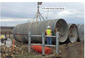
Figure 2: Steel Pipe for Cased Application, 20-ft Sections with Two Brush Bands per Section
