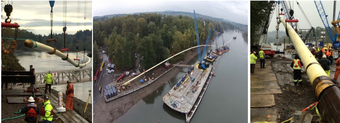
Figure 12a, b, c: Lineup of Pipe in Preparation for Pull-back; Complete Line Ready for Pull-back; Pull-back Commencement by Insertion into
