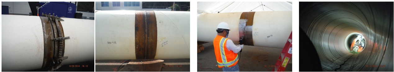
Figure 10a, b, c, d: Joint alignment for Butt Welding, Completed Butt-welded Joint; Surface Grinder Used for Substrate Preparation for External Joint Completion, Surface Preparation for Internal Joint Completion
