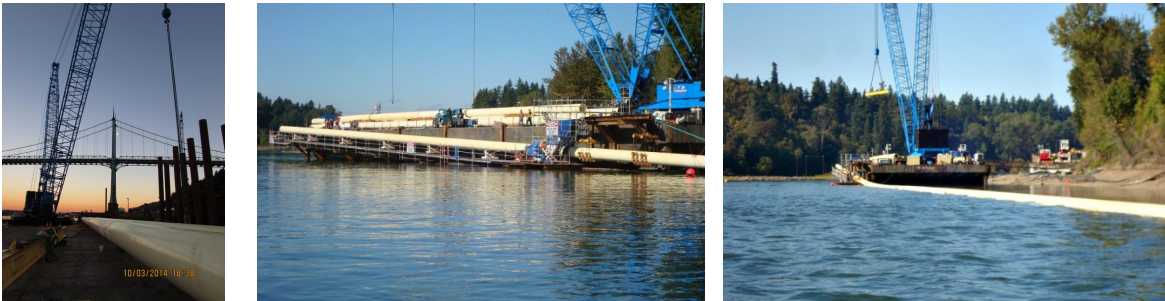
Figure 9a, b, c: 240-ft Welded Segment of Steel Pipe, Transportation of 240-ft sections by Derrick Barge, Final Joint Assembly Prior to Pull-in
