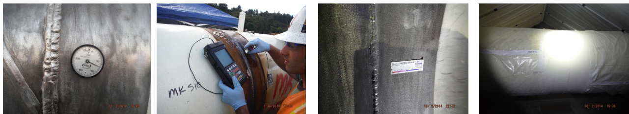
Figure 11a, b, c, d: Ambient Temperature Conditions, Surface Temperatures, Testex Tape for Anchor Profile Testing, Completed Joint Coating
