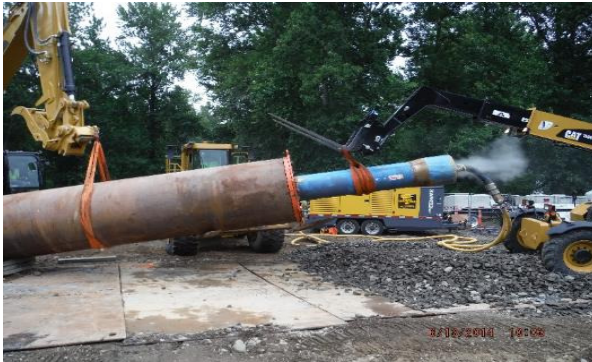
Figures 8a, b: Pipe Ramming of 60-inch Conductor Casing; 840,000 lb HDD Rig
