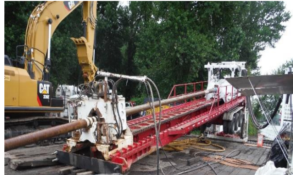
Figures 8a, b: Pipe Ramming of 60-inch Conductor Casing; 840,000 lb HDD Rig
