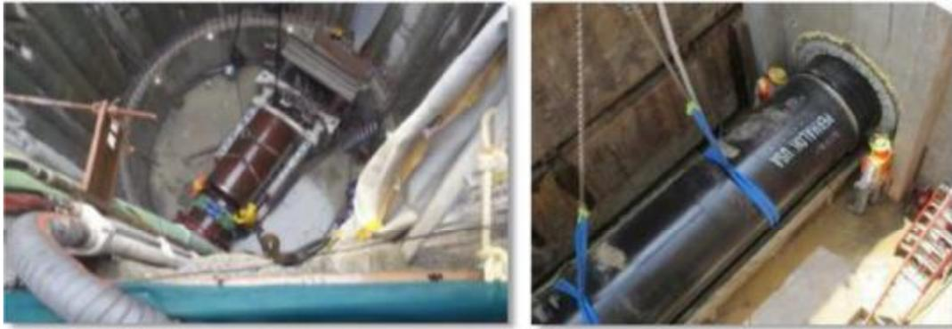
**Figure 3. Microtunneling**
