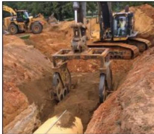
**Figure 9: CSS Being Compacted with Roller**
