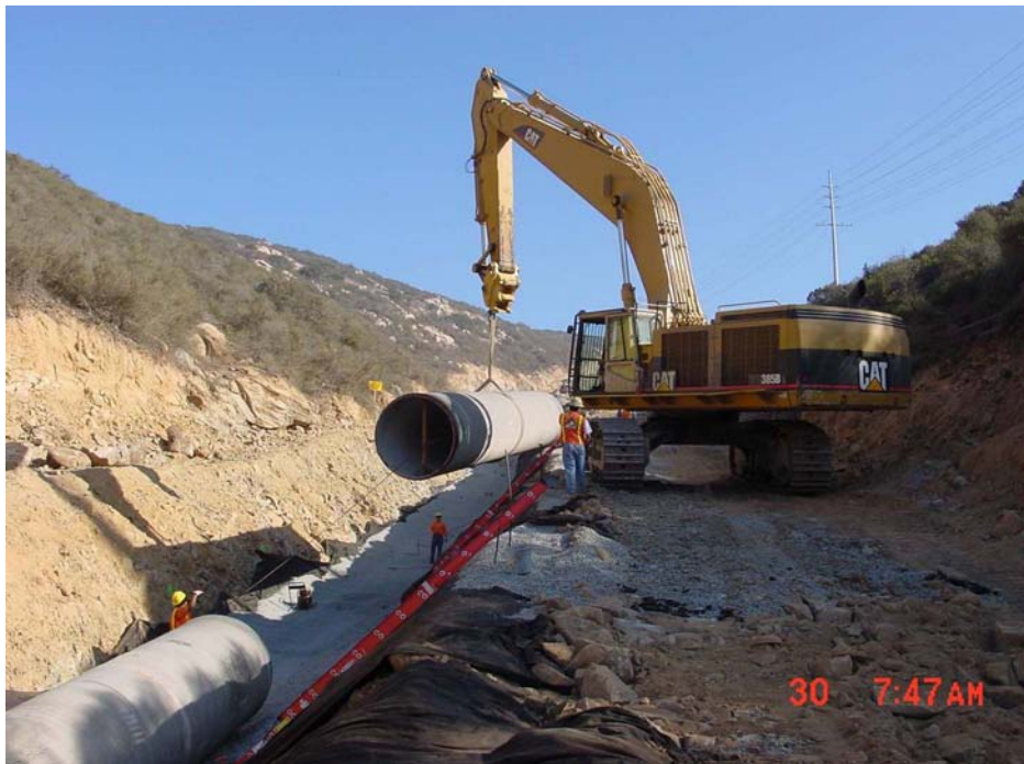
Figure 7. Installation of 66-inch diameter CCP
