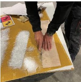
Measure the area of the grout to be covered and add ½" per side. Mark and cut the woven FRP sheeting to size. It is recommended to cut the FRP sheet into four separate pieces.
