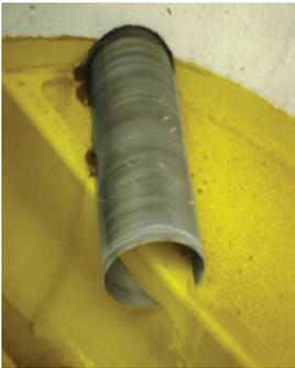
Establish the alignment and elevation of the new connection that is to be made. Core an opening through the outside of the manhole into the main channel. It is recommended to make the opening 2" larger than the OD of the new connecting pipeline. Coring bit should be long enough to reach the main channel (be ½ the inside diameter of the manhole plus the manhole wall thickness.) If a coring machine is unavailable, create a rough core using a grinder with a masonry blade and a roto hammer.
