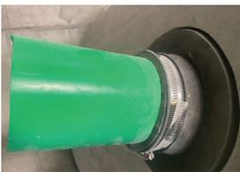
Inspect all coated surfaces and ensure that the area is completely sealed with the gelcoat coating. If correctly sealed, tighten the boot and return the manhole to service.
