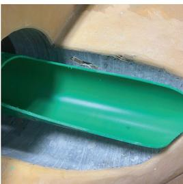
Using an angle grinder with a cut off blade or a keyhole saw trim the PVC pipe along the marked area of the top and end of the pipe.
