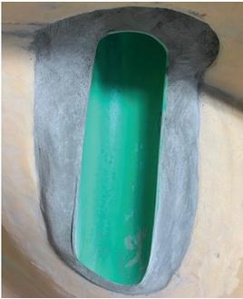
Inset the PVC pipe into the manhole and place a spacer under the pipe to create a consistent flow line and create an annular space for the grout. On the inside end of the manhole shelf place a piece of cardboard against the channel and secure it with duct tape to dam the ends of the cavity for grout. Install the boot on the outside of the manhole. On the inside of the manhole pack grout around the PVC pipe and finish the top of the grout with a damp sponge. Allow the grout to dry.
